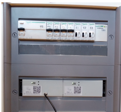
SPM and PMC measuring devices supporting the operation of smart energy networks.
